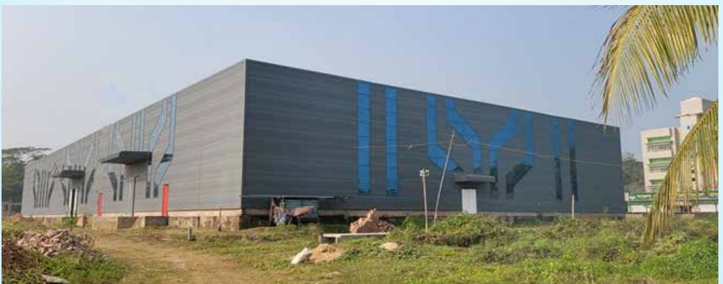
Single Storied factory shed at Noakhali
