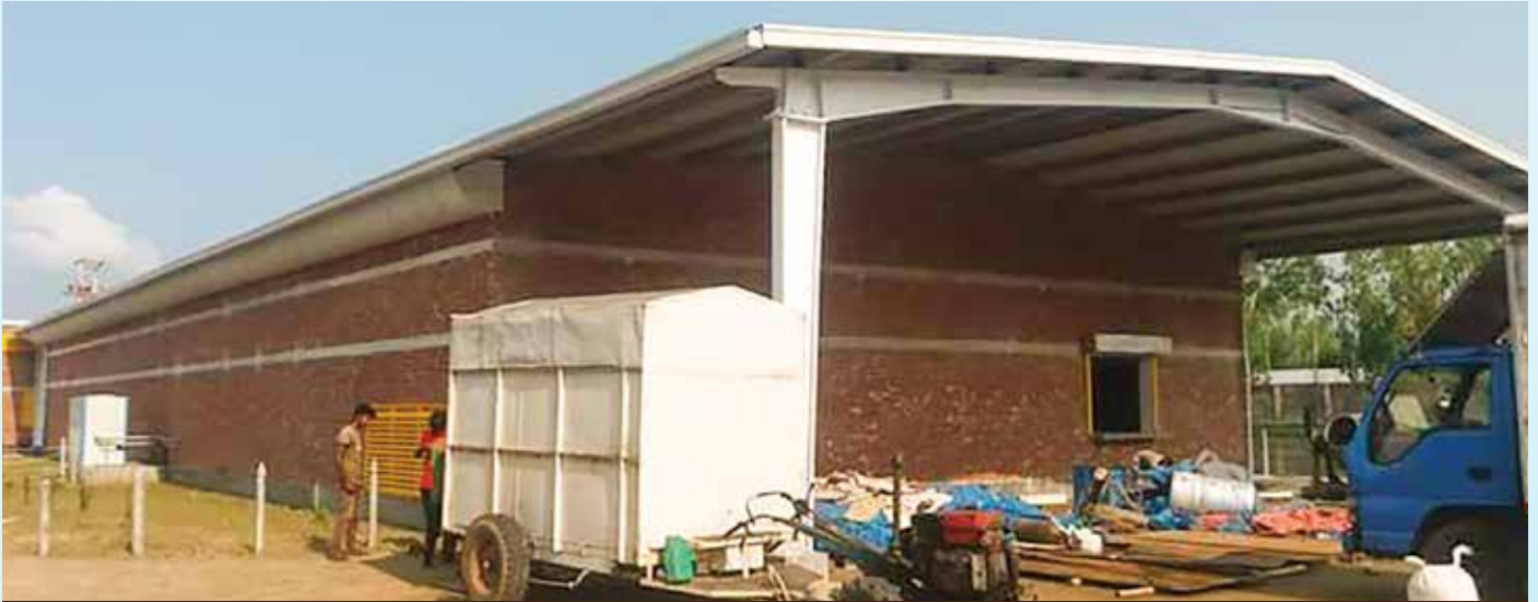
Single Storied Hatchery shed at Bogura
