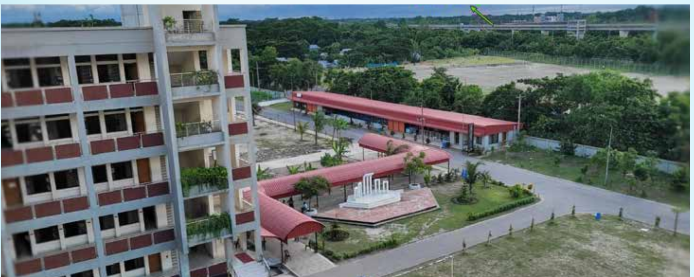
Single Storied waiting Room shed and Walkway at PCPSC, Zajira
