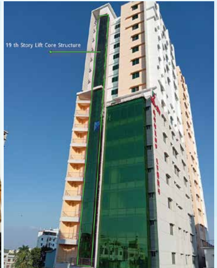
Steel Lift Core Structure at Rajshahi
