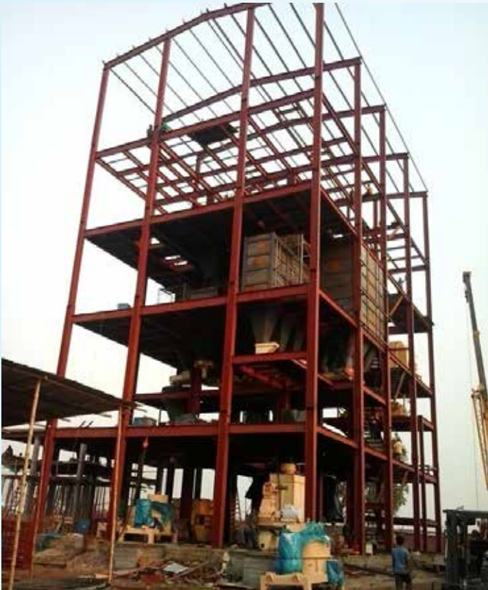
Feed Mill Structure at Bogura
