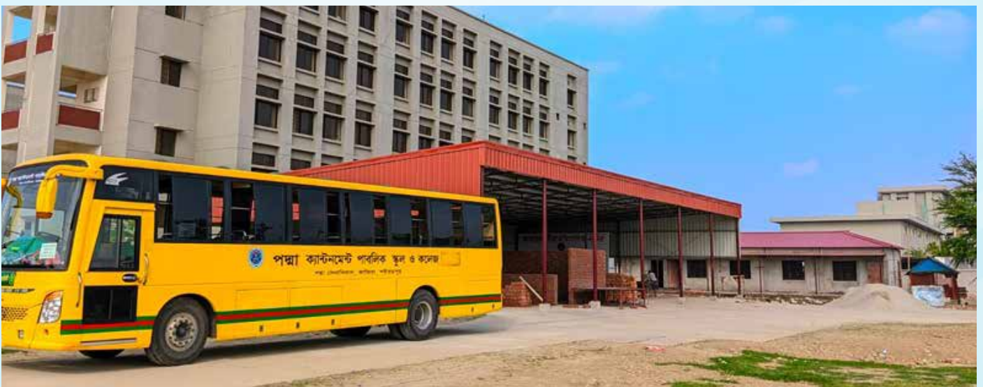
Single Storied Car Parking shed of Padma Cantonment Public school and College
