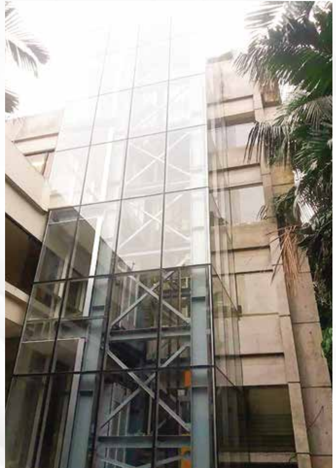
4-Storey Lift Core of BAEC at Dhaka
