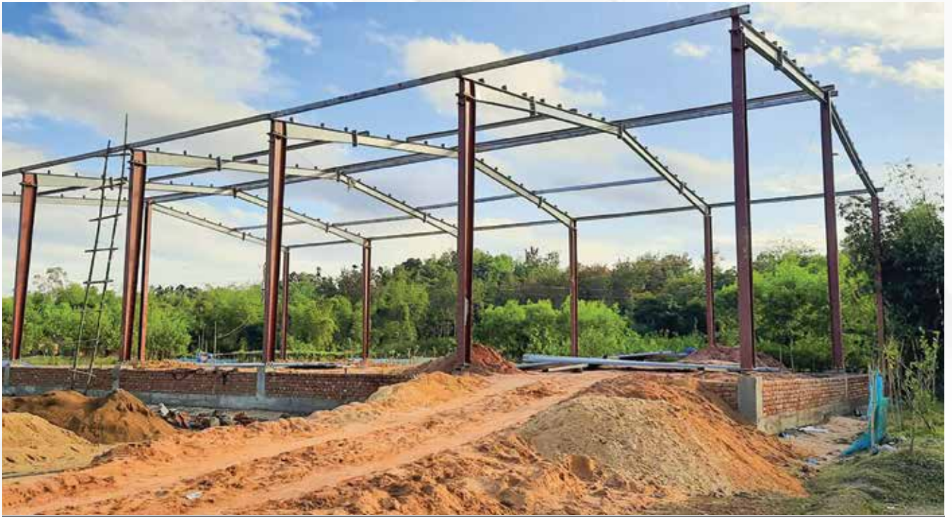
Single Storied Brick Filled Shed at Sylhet
